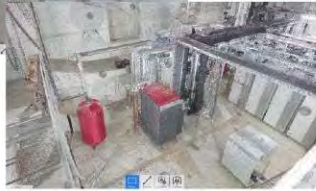
BLK360 point cloud
