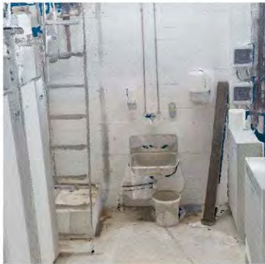
Details from the heating room 3D mesh
