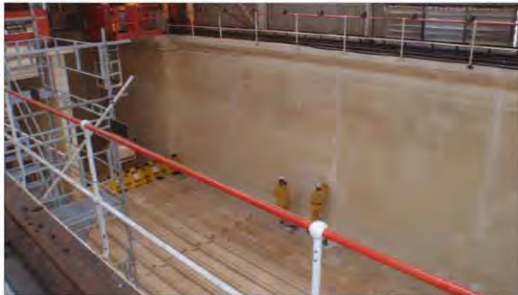
Pond 1 at Chapelcross Nuclear Facility. Pond had been decommissioned, emptied, and decontaminated in preparation for Care and Maintenance phase.
