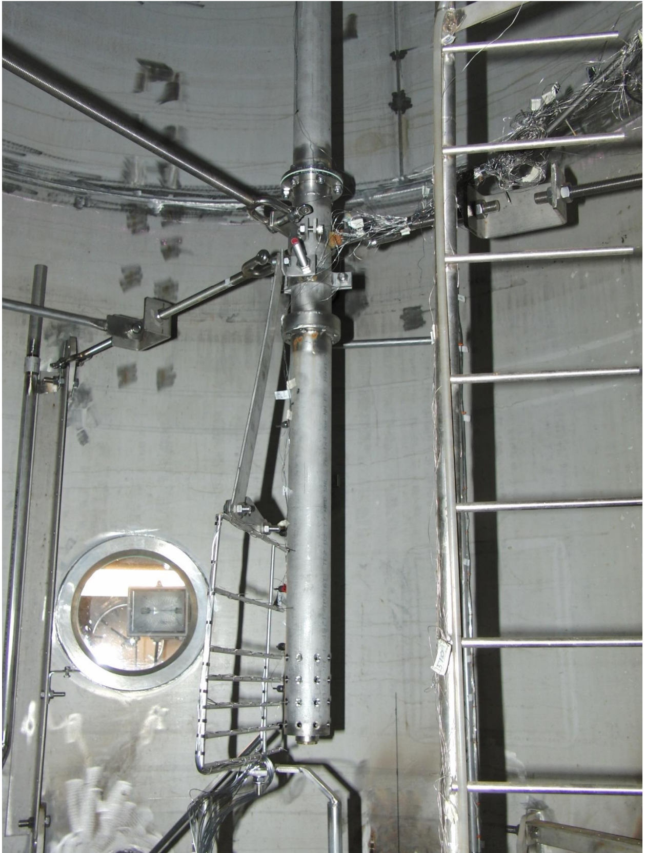
Lower part of the sparger pipe.
