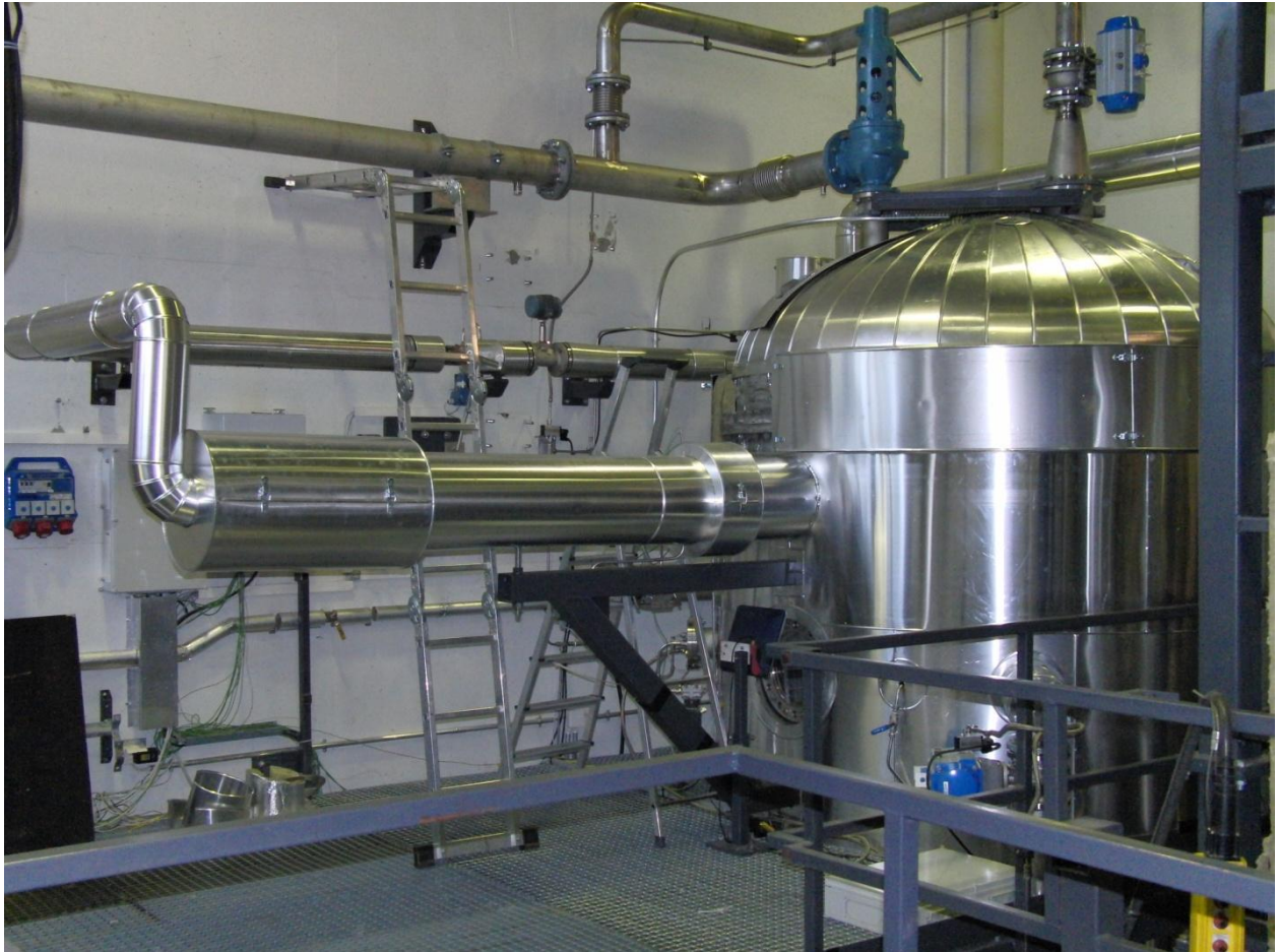
Mineral wool insulated dry well compartment and steam line.
