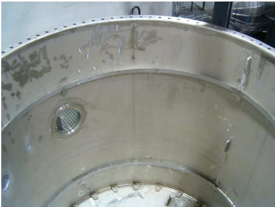
Drain gutters on the dry well inner wall on two elevations.
