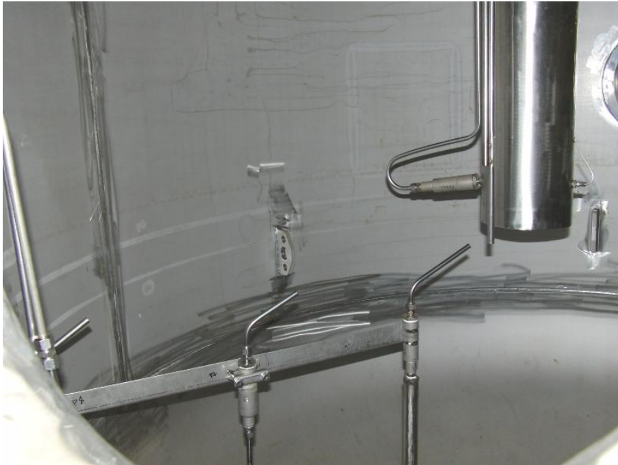
Pressure (P1, P5, P7 and P8) and temperature (T1 and T5) measurements at the blowdown pipe outlet.
