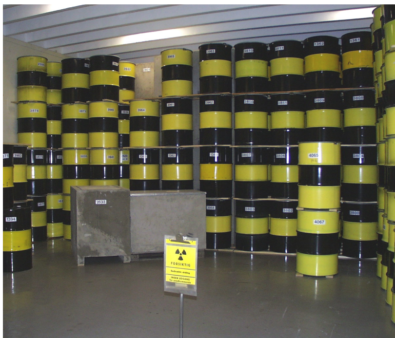
Figure 5. Intermediate storage of drums in a heated storage building at Kjeller in Norway.
