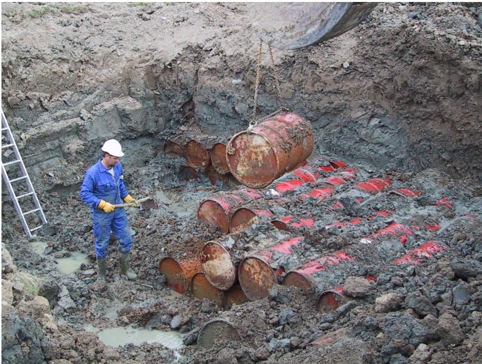
Figure 9. Retrieval of disposed drums at Kjeller .
