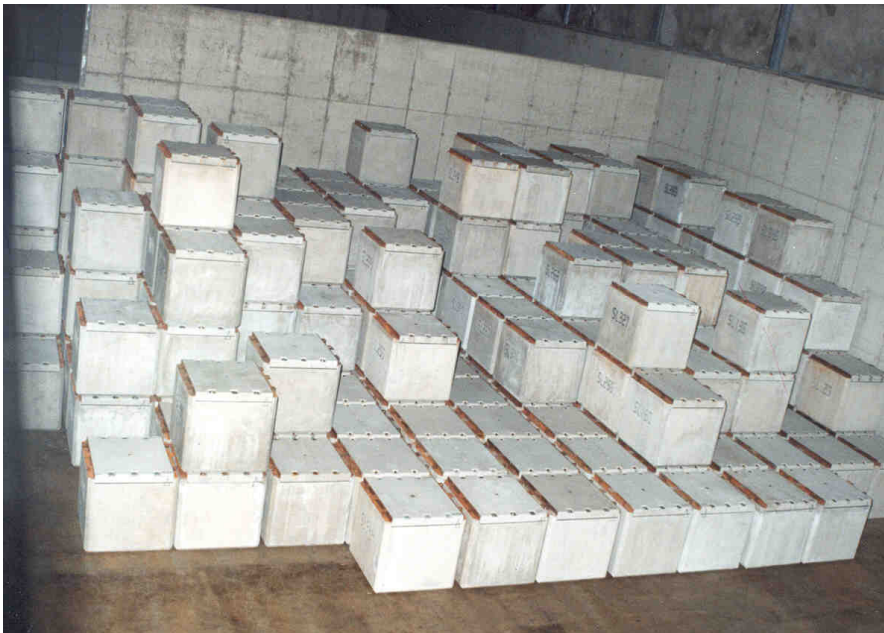
Figure 6. Intermediate storage of drums and concrete containers in rock vaults at Studsvik in Sweden.
