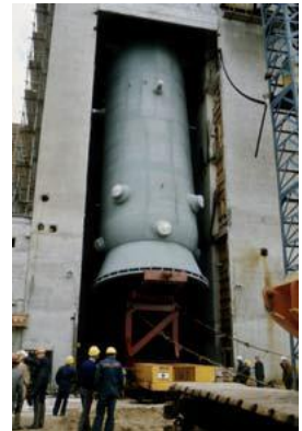
Reactor pressure vessel installed in B2, photo: Barsebäck Kraft
