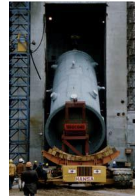
Reactor pressure vessel installed in B2, photo: Barsebäck Kraft
