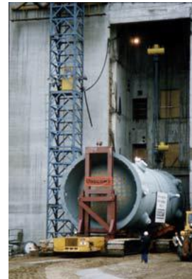
Reactor pressure vessel installed in B2, photo: Barsebäck Kraft
