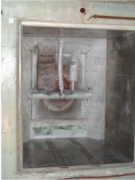
Figure 9 Thermal column with lead nose exposed
