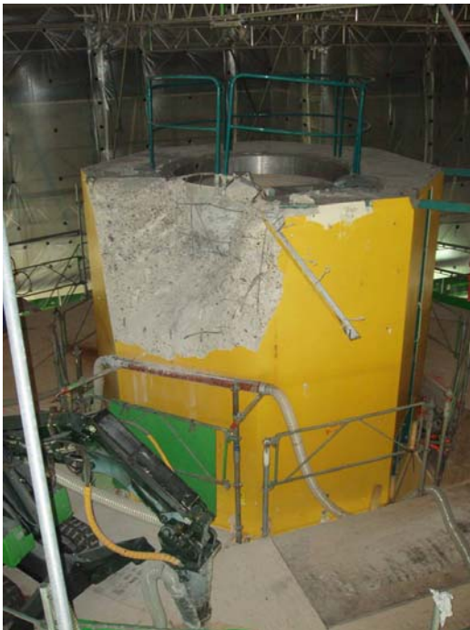
Figure 14 Start of demolition from a platform
