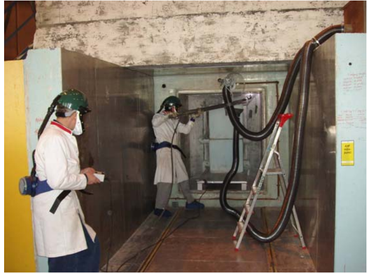
Figure 10 Plasma cutting of the lead nose
