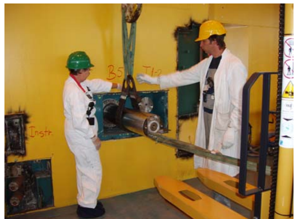
Figure 5 Removal of a beam tube (plug)
