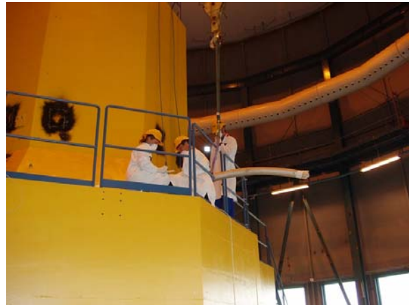
Figure 4 Removal of an "S" tube
