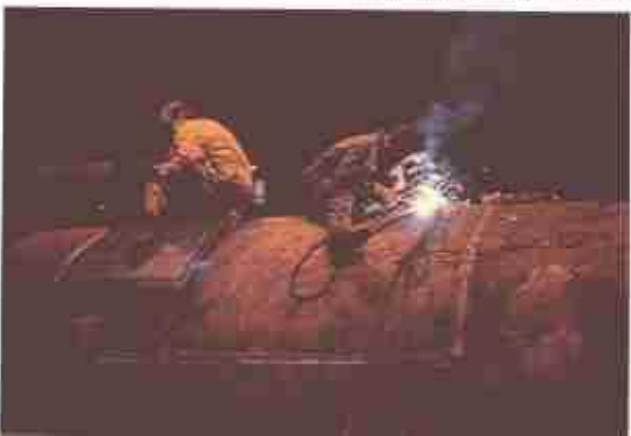
Sealing a tank containing aircraft debris.
