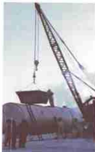
Crate lowering a crane with 28,000-gallon tank prepositioned to loading it with debris-laden snow and ice.
