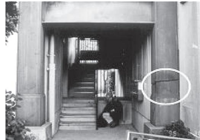
Ashiyahama apartment building (Kobe). Brittle fracture of steel box-section columns in a modern 51 buildings, situated on the fracture line.
