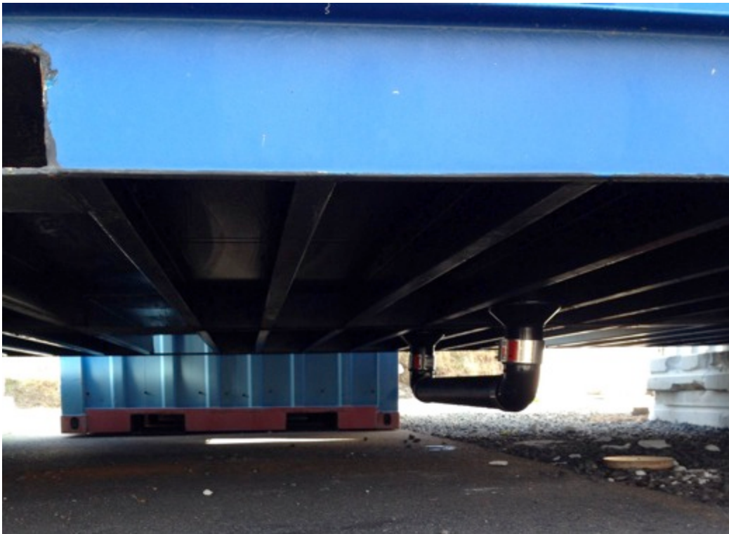
Figure 66 The connecting pipe between the floor drains in the two rooms (fire and non-fire room).
