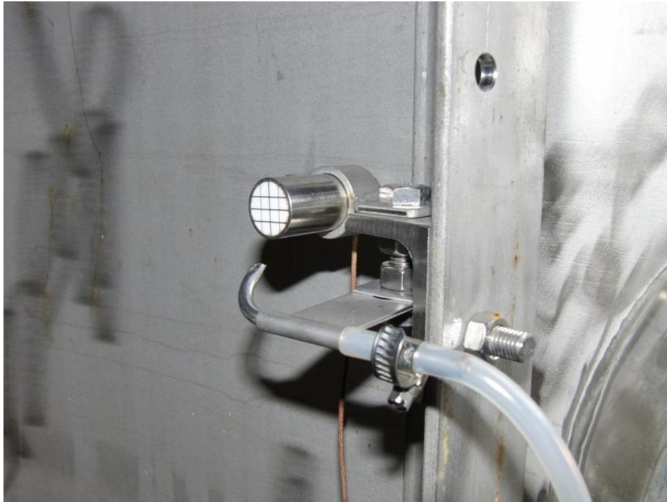
Close-up view of the ultrasonic transducer installed in the wet well compartment.
