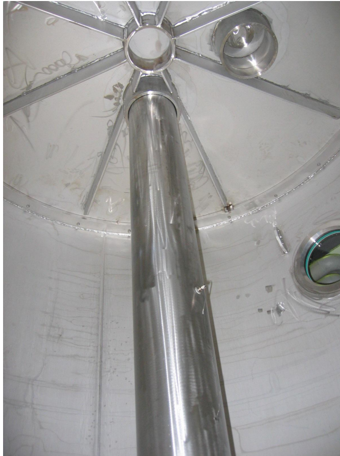
Blowdown pipe and intermediate floor.
