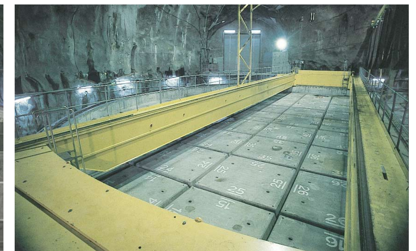
View over top of silo
