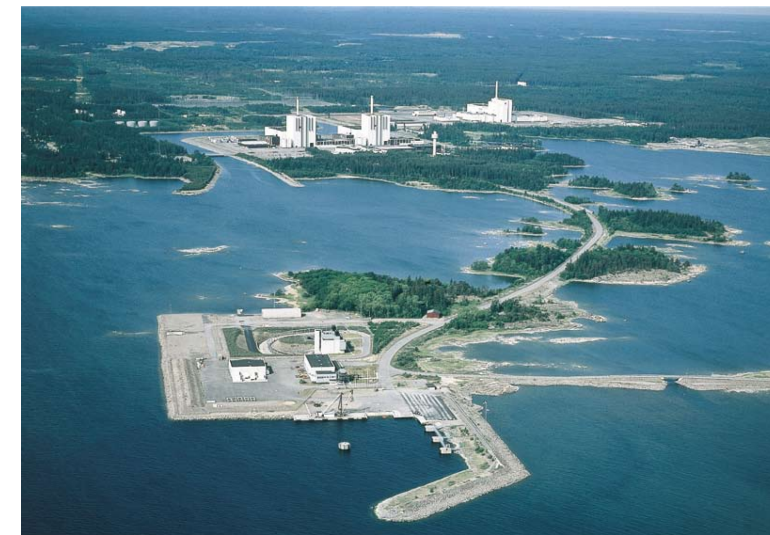
View of the surface part of SFR (Forsmarks NPP is in the background)
