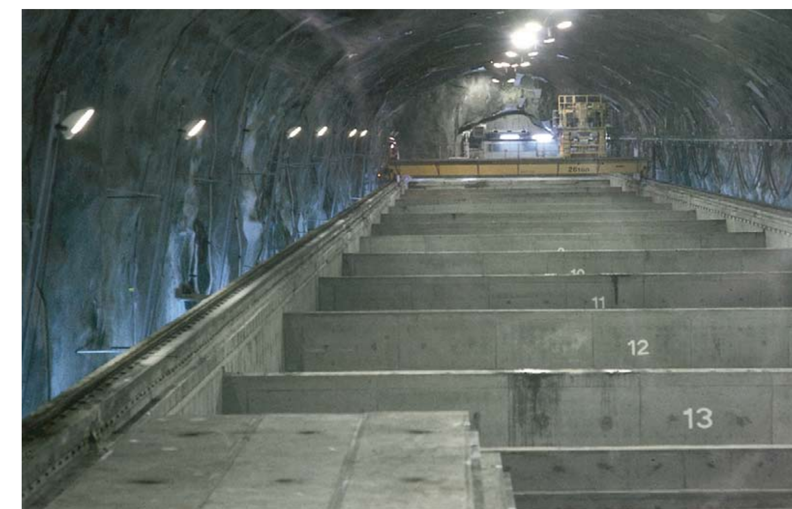
Rock vault for intermediate-level waste
